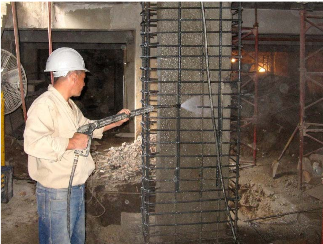
Fig 6: Surface preparation of section enlarged columns
