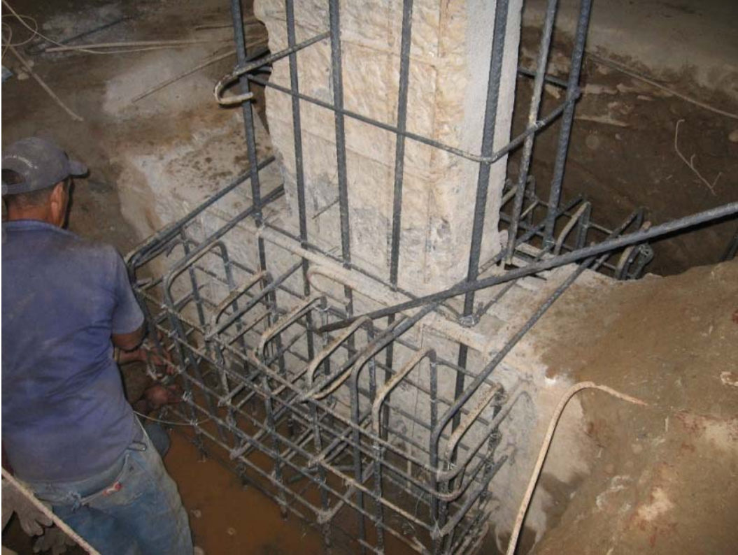
Fig.3: Foundation reinforcement for section enlarged columns
