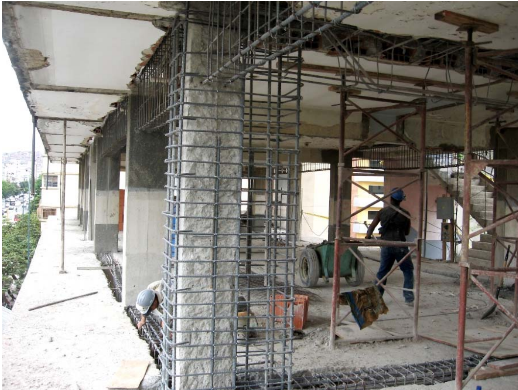
Figure 9: Detail of new steel reinforcement in section enlarged columns and beams
