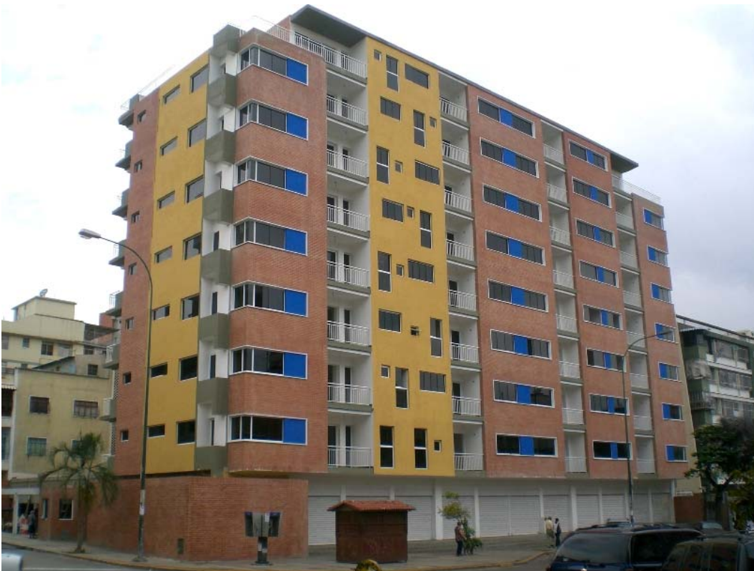
Fig 2: Building appearance after refurbishment
