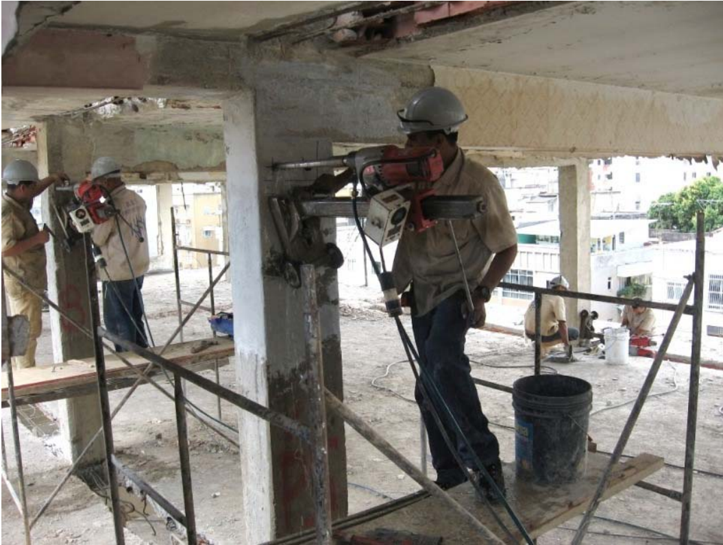
Fig 5: Drilling columns for placing the new reinforcing steel of beams
