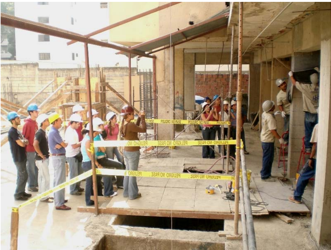
Fig 8: Civil engineer students in a guided visit to the job site
