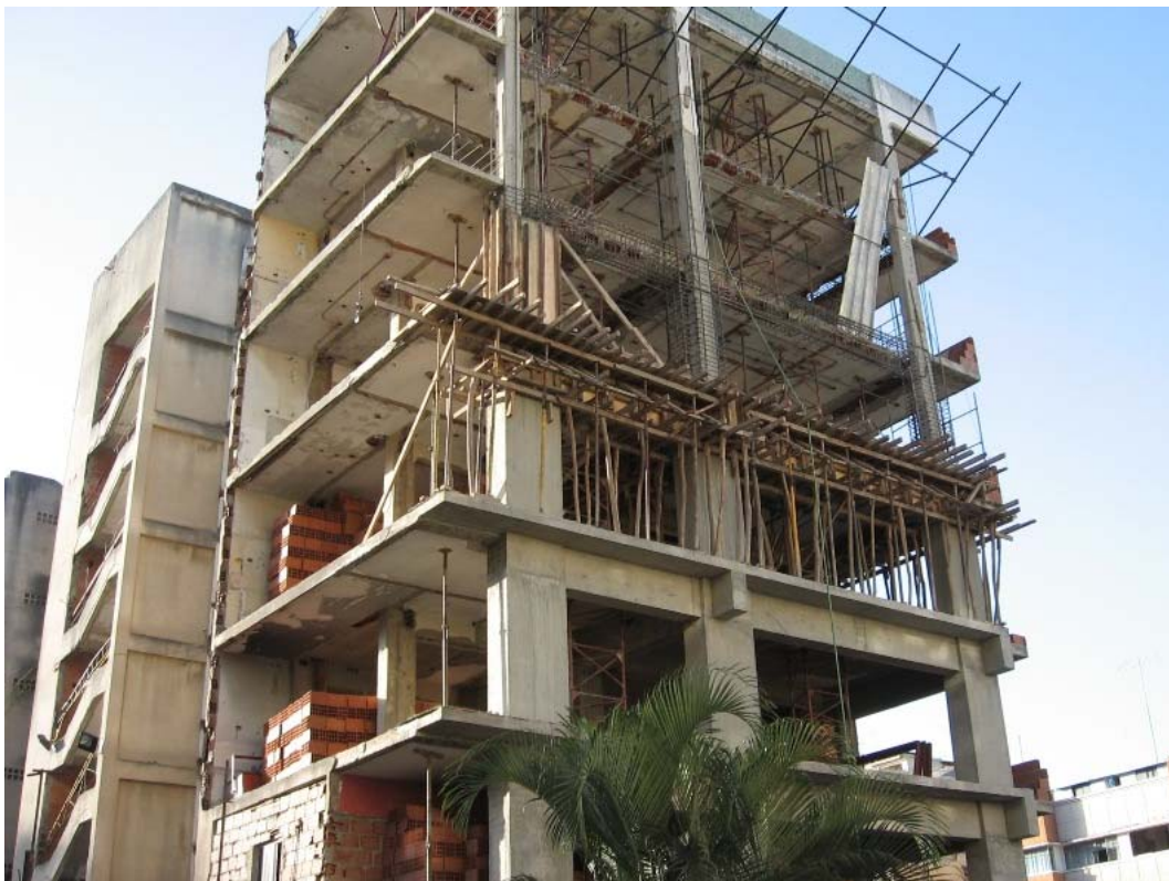
Fig 10: Retrofitting in progress
